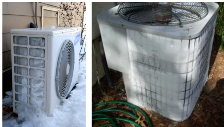
Figure 6: Impact of Snow Accumulation (left) and Ice Formation (right) on Electric Heat Pumps
