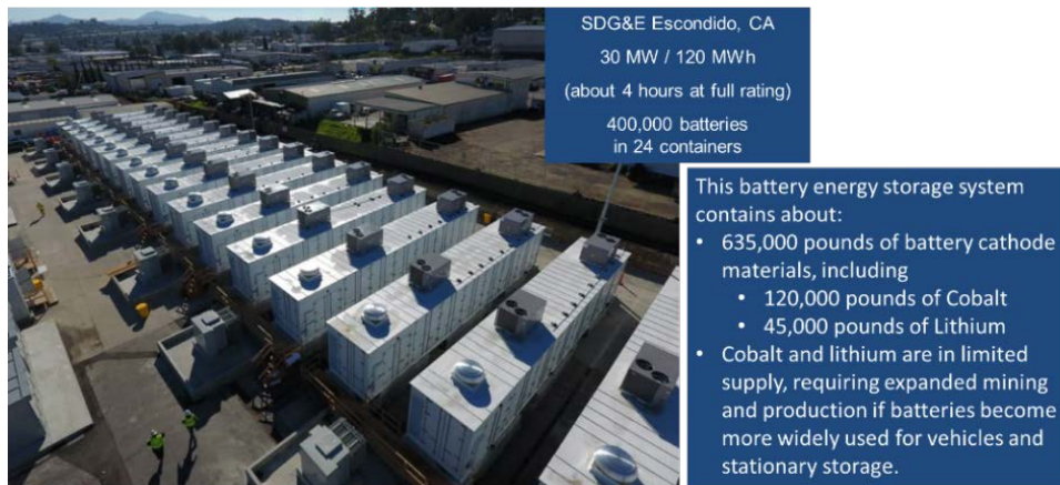
Figure 12: Example Large-Scale Battery Energy Storage System
